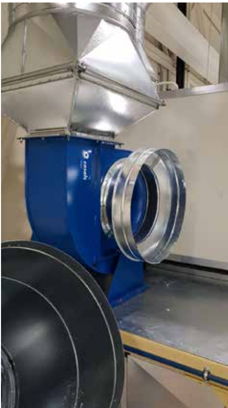
Medium pressure extraction in automotive factory with ATEX environment MBX
