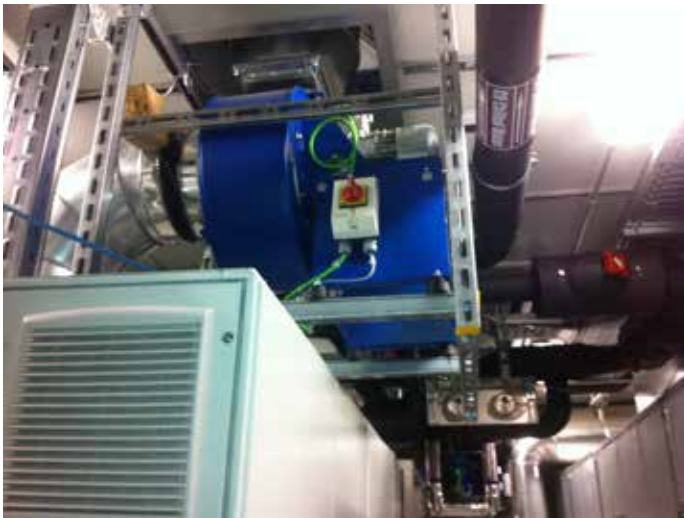
Jaguar Land Rover factory, AVL Powertrain Technical Center, Ansty Business Park, Coventry (United Kingdom) MBX ATEX with explosion-proof enclosure for explosive atmospheres class Ex-d.
