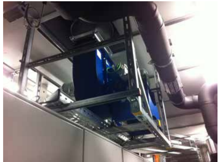
Jaguar Land Rover factory, AVL Powertrain Technical Center, Ansty Business Park, Coventry (United Kingdom) MBX ATEX with explosion-proof enclosure for explosive atmospheres class Ex-d.
