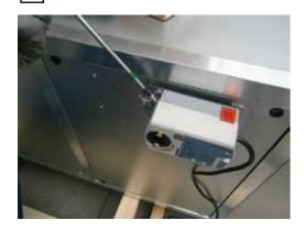
Operate the release button and bring the end of upward stroke, in this way the white wire will go to close the by-pass while the black wire going to open it.
